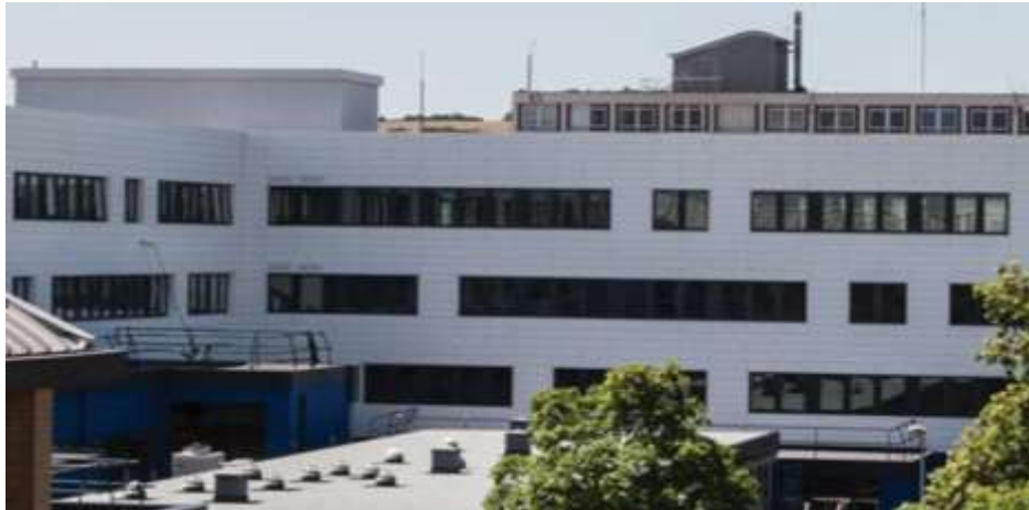
Figure 12: Before and after photos of cladding installation at RAL site, Didcot, Oxfordshire.
